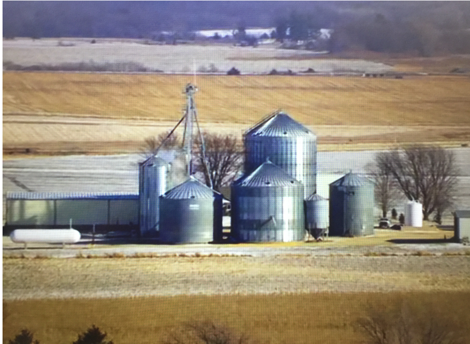
Figure 2. The Soules farmstead shows viewers a modern grain facility, complete with a propane tank and tower dryer. The farm also shows their machinery storage barn and shop equipment.
